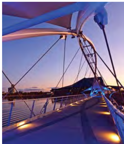
Signature Pedestrian Bridge
