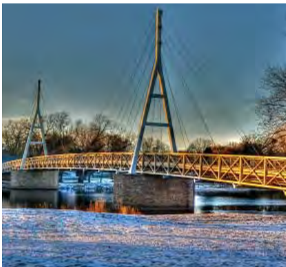
Signature Pedestrian Bridge
