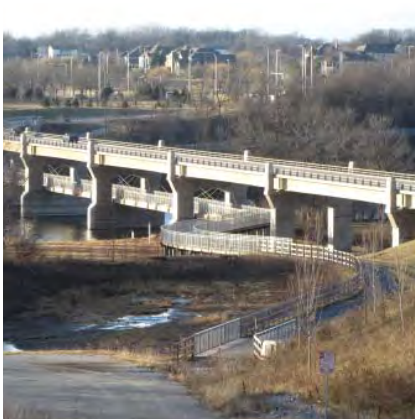
Red Gate Rd Bridge Trail Connection
