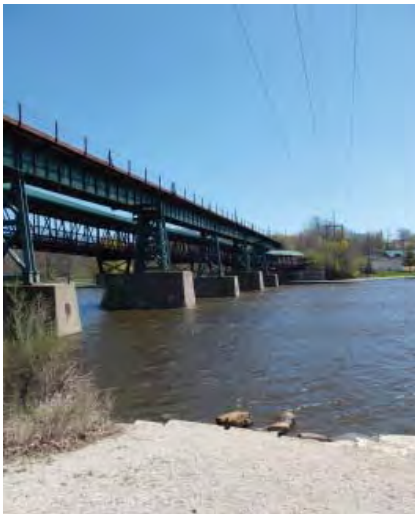
Union Pacific Railroad Bridge
