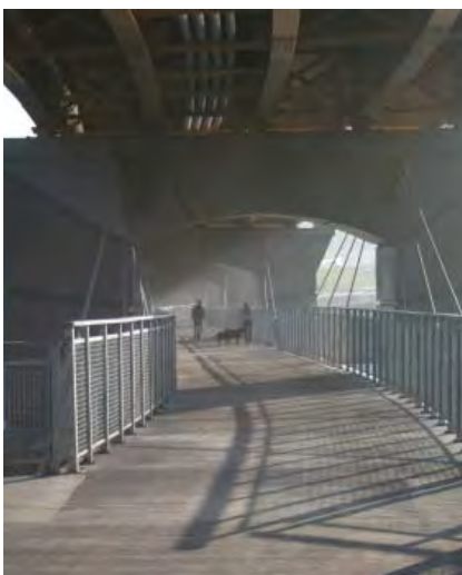
Red Gate Rd Pedestrian/Bike Bridge
