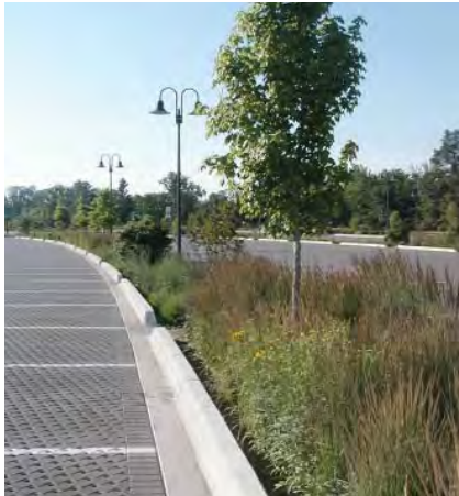
Permeable Paving/ Bioswales
