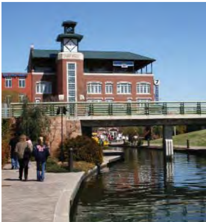
Under Bridge Connection
